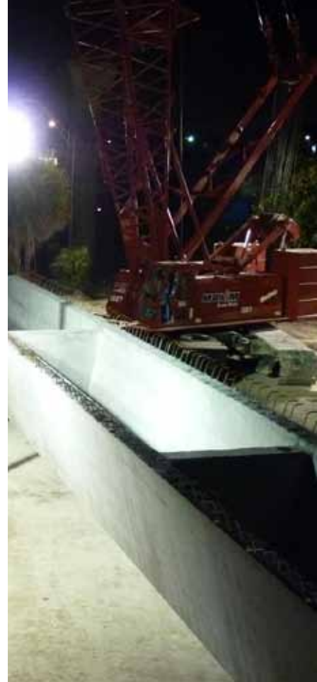
277,000 pound Precast Beam
