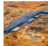
Thyssen-Krupp Steel Mill Calvert, Alabama
