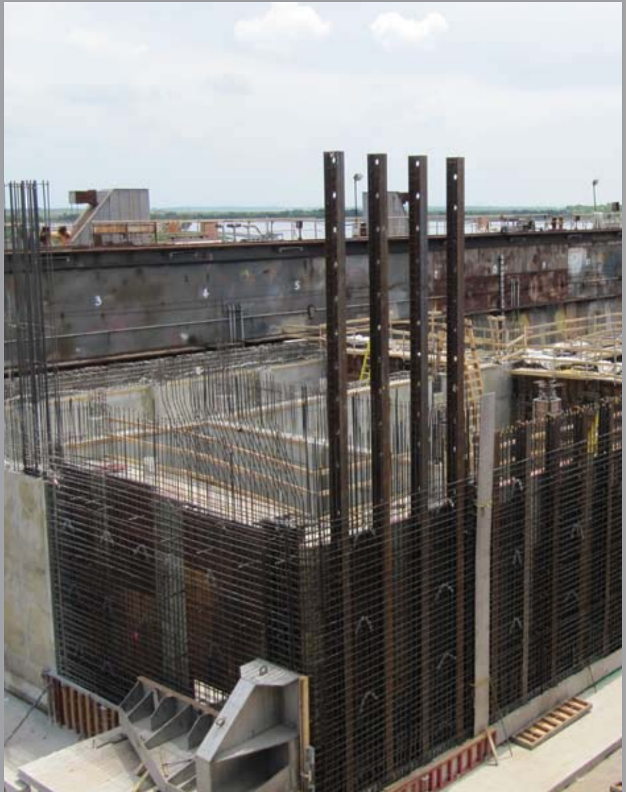
Concrete Swing Gate, Inner Harbor Navigation Canal Surge Barrier - Under Construction
